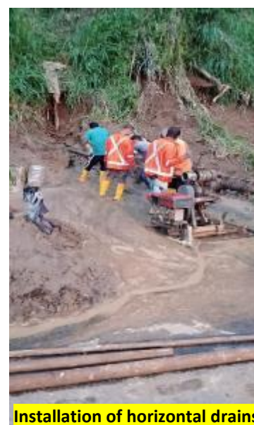
Discharge measurements from horizontal long drains during rapid mitigation measures before reopening the road:
