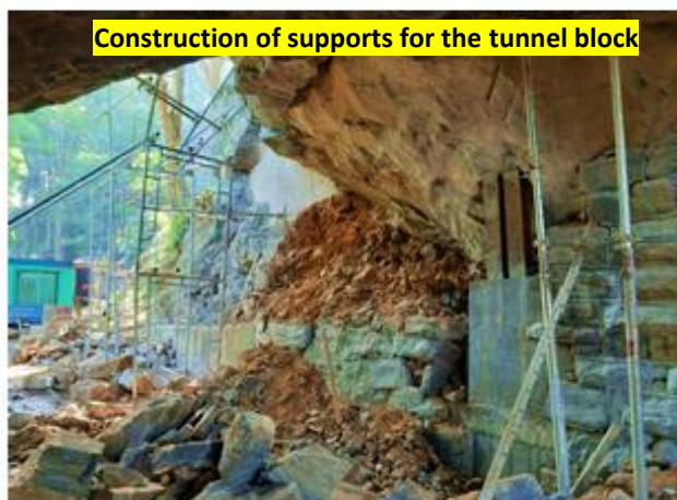
Demolishing of existing wall
