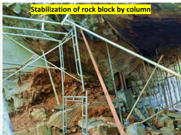
Construction of supports for the tunnel block
